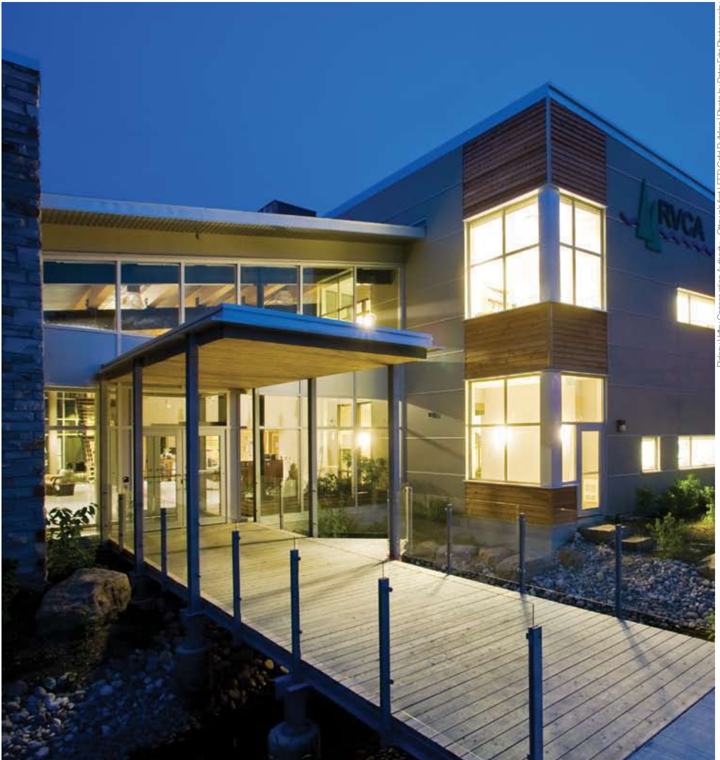
Rideau Valley Conservation Authority – Ottawa's first LEED Gold Building | Photo by Peter Fritz Photography
